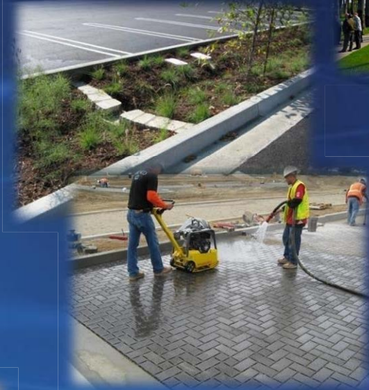
Los Angeles Zoo Parking Lot - Vegetated bio-swale & Permeable pavers
