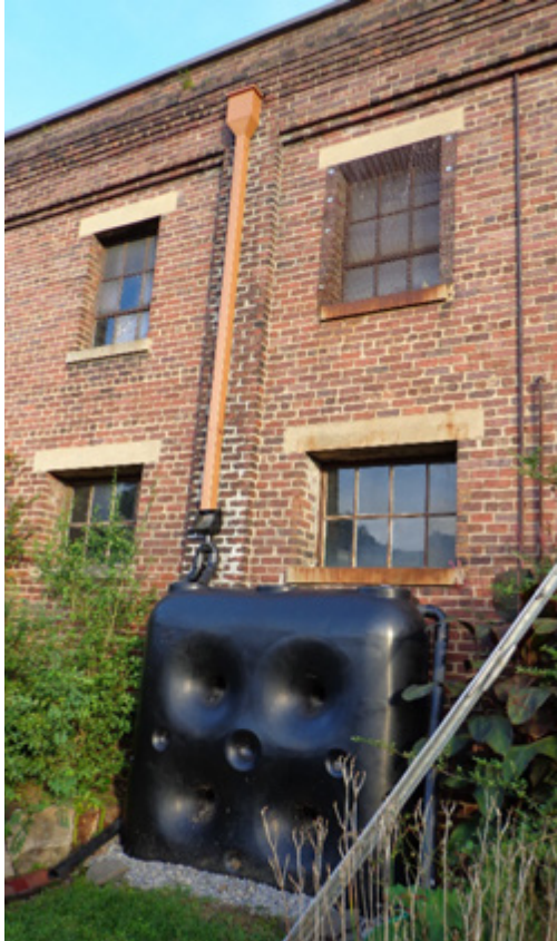
Rainwater Harvesting & Reuse
