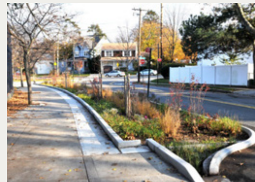
STORMWATER GREEN STREETS / BUMPOUTS
