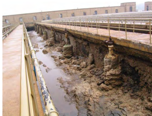
Separate Centrate Treatment Aeration Tanks
