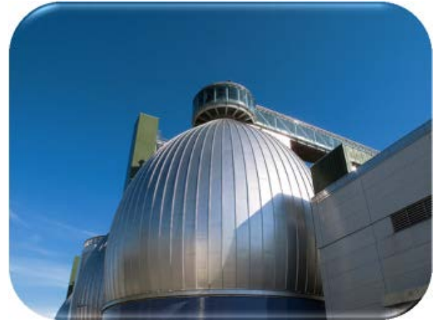
Anaerobic Digester Newtown Creek WWTP, NYC
