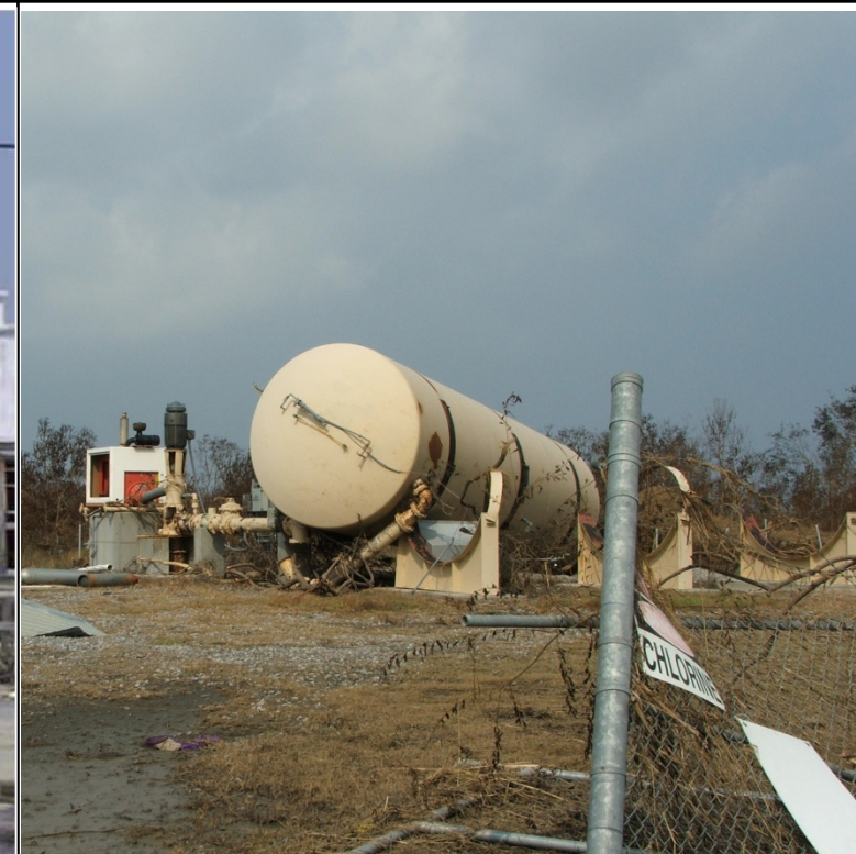
Cameron, LA, water storage tank, destroyed by Hurricane Rita, 2005 (R. Reeves, LRWA)
