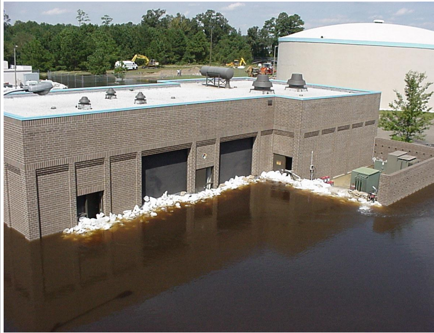
Greenville Utilities, NC - Hurricane Floyd, 1999 (S. Porter)
