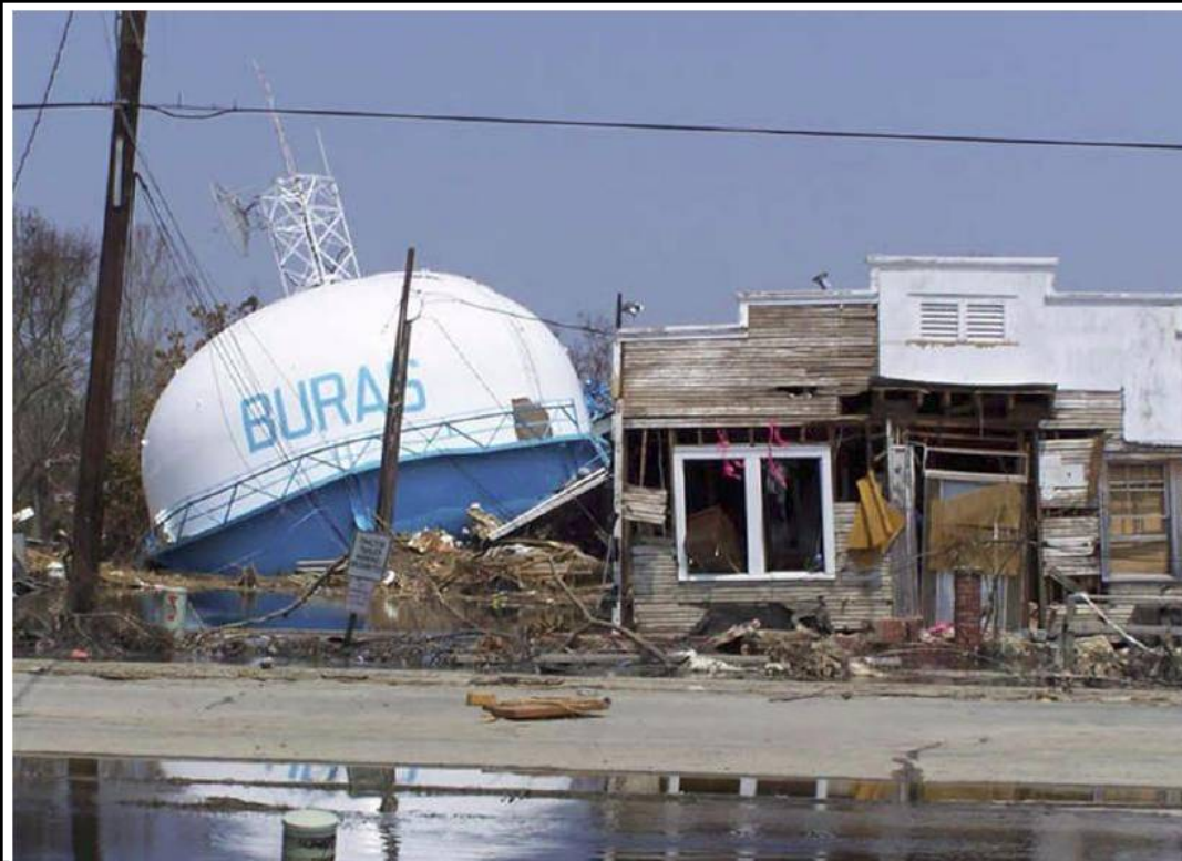
Buras, LA, elevated water storage tank, destroyed by Hurricane Katrina, 2005 (C. Carlson, LA Dept of Health and Hospitals)
