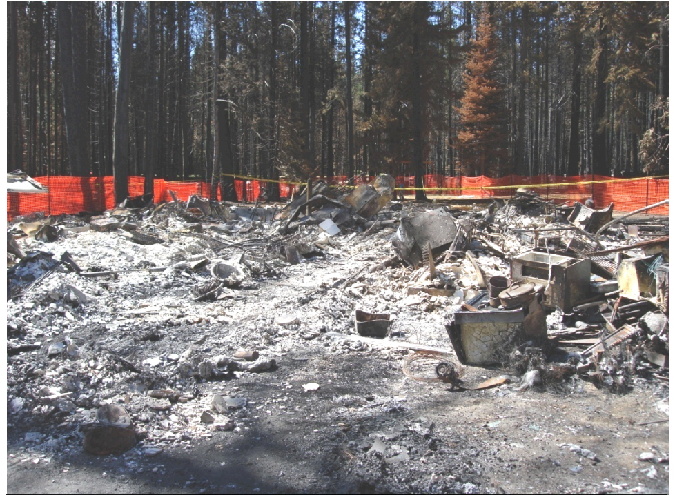
Lake Tahoe 2007 Angora Fire - Burned house with open sanitary sewer lateral (Photo: Paul A. Sciuto, STPUD)
