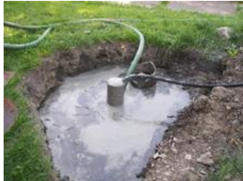
Leaking 75- year- old, abandoned gas well in NY state.
