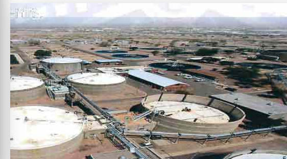
Roger Road WRF Decommissioning
