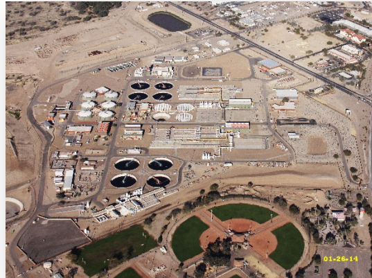
Tres Rios WRF Upgrade & Expansion
