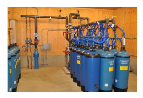
Loaded media and canisters can be removed offsite and disposed of safely.
