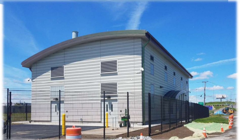
West Side Pump Station (40 mgd) $x Million
