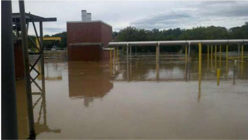
BJC WWTP inundated by floodwaters (DEC photo)
