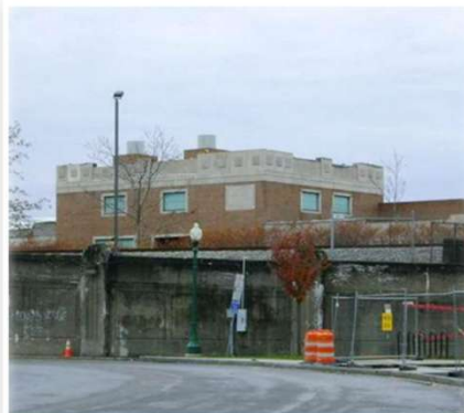
View of Clinton CSO Storage Facility West Chamber from West Jefferson Street November 2013
