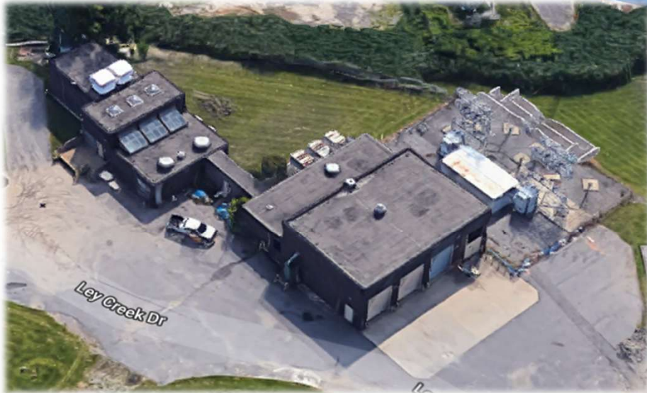
Ley Creek Pump Station (20 mgd) $X Asset Value
