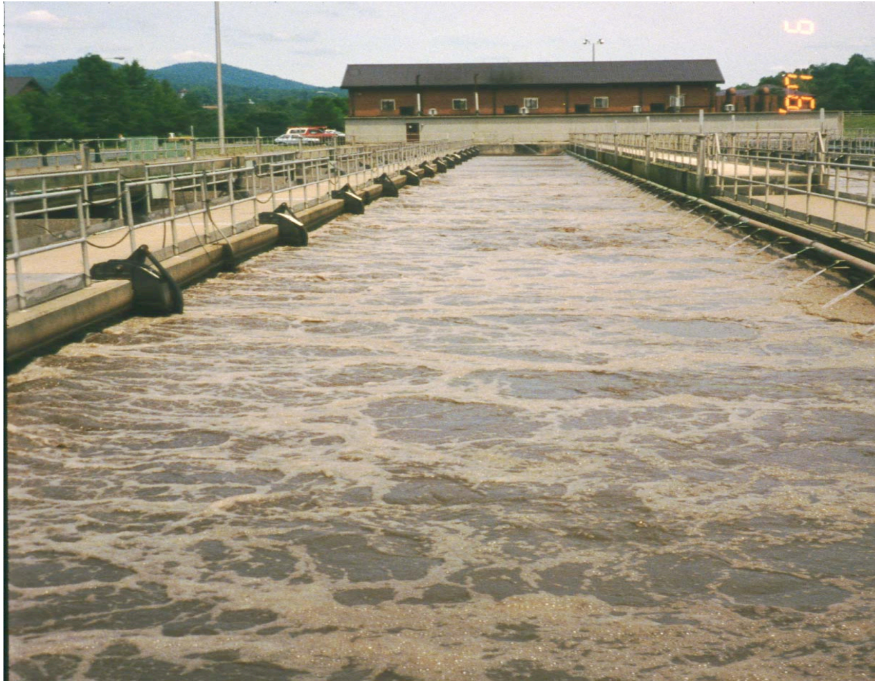
Aeration Basin Before Modification Moore's Creek WWTP, Charlottesville, Virginia
