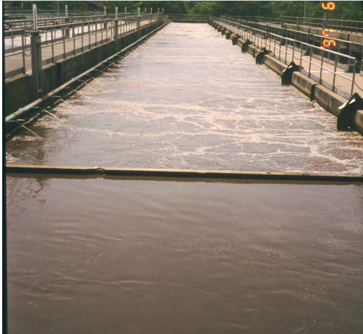
Aeration Basin After Modification Moore's Creek WWTP, Charlottesville, VA
